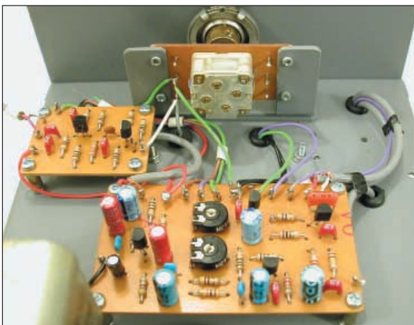
The Buffer Amplifier wired to the Regenerative Radio (Part 3) and the tuning capacitor p.c.b.s.
